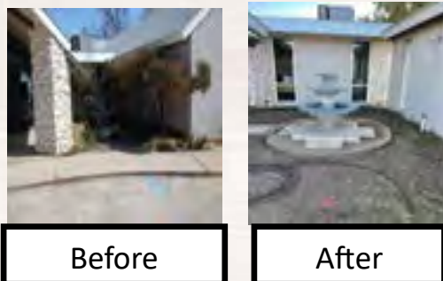
The Fountain was repaired by Ricci Bickle and his brother.
